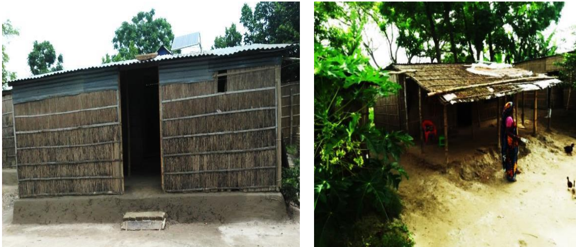
Photo 1 Poor structure of dwelling houses of char children
